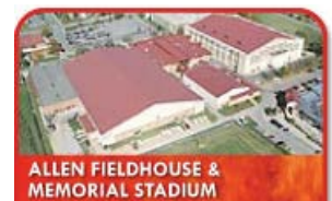
The university requested that Poole Fire Protection draft the
